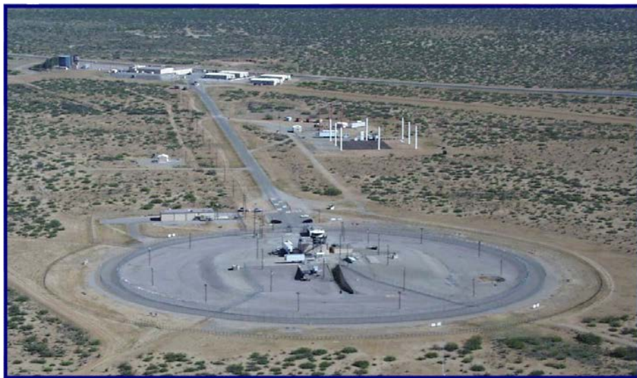
Fast Burst Reactor Survivability, Vulnerability and Assessment Directorate(SVAD) Nuclear / DEW / E3/ Environmental Facilities and Capabilities. 29 July 2009. Approved for Public Release.
