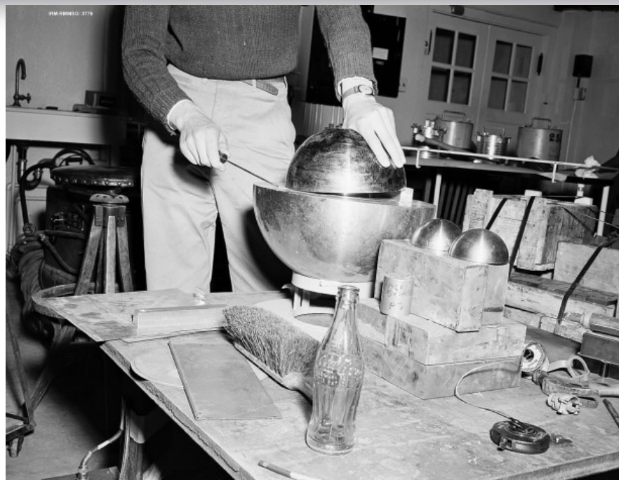
A recreation of the criticality experiment that Slotin conducted. Image from http://nerdist.com/tickling-the-dragons-tail-the-story-of-the-demon-core/
